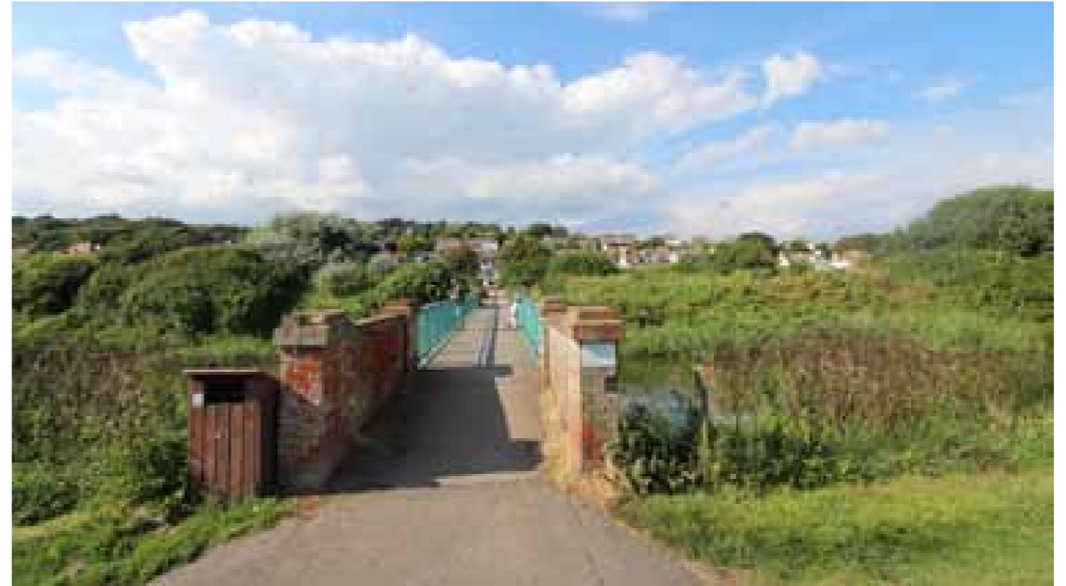
fig. 26 View looking north along Sea View Bridge
