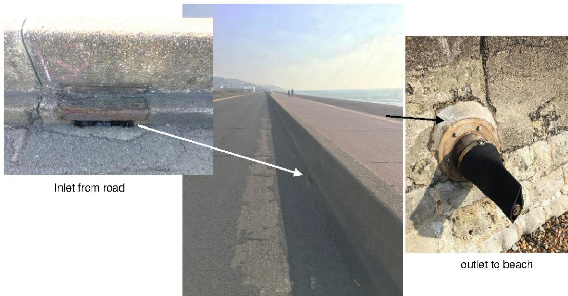
Figure 3.3 – Existing road drainage along Princes Parade.
