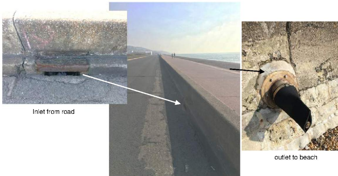
Figure 3.3 – Existing road drainage along Princes Parade.
