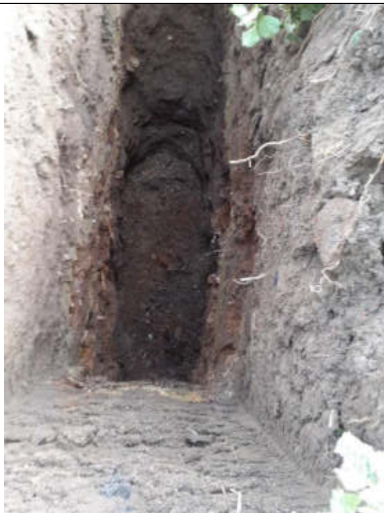
Plate 96: TP112 finished excavation.
