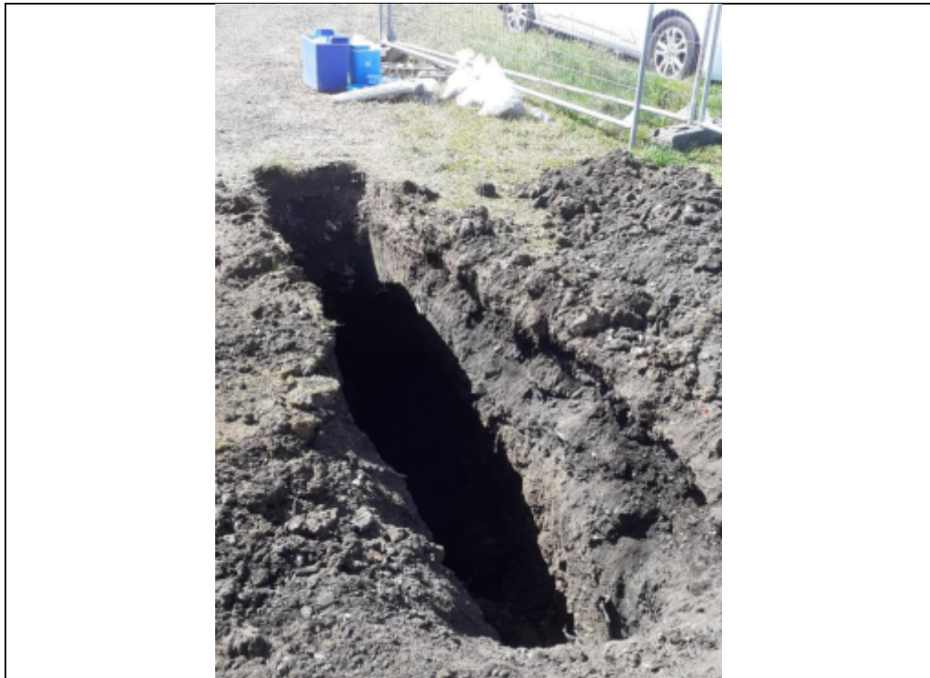
Plate 275: TP131 finished excavation.
