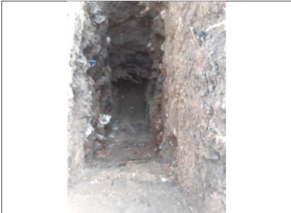
Plate 287: TP132 finished excavation.
