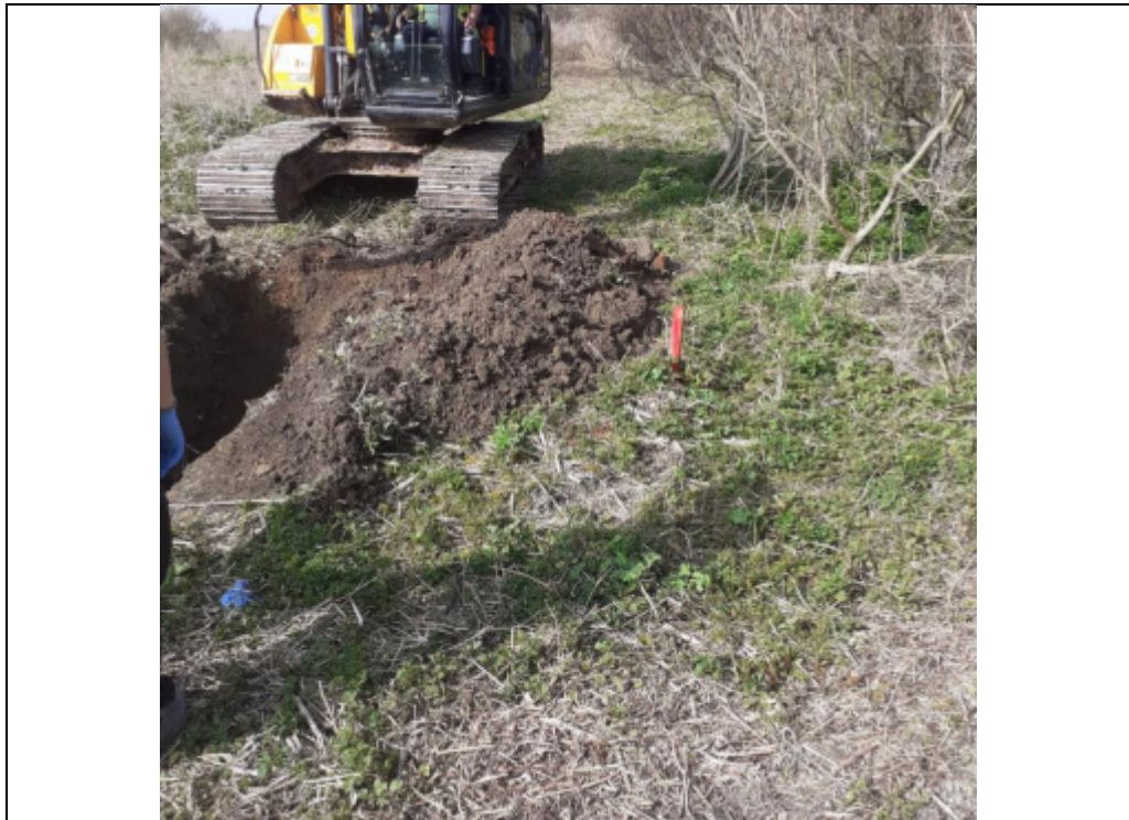
Plate 149: TP119 ranging from ground level to 0.6 m bgl.
