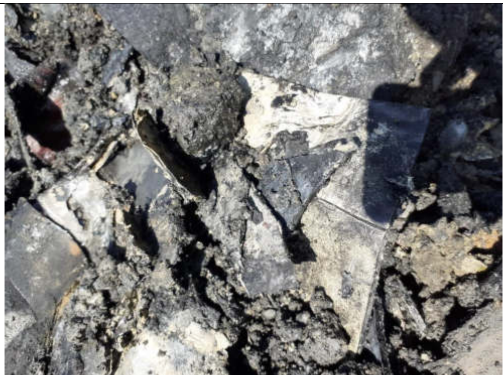
Plate 224: TP126 potential asbestos material.
