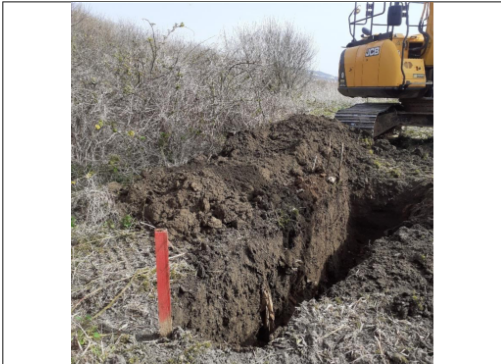
Plate 141: TP118 ranging from ground level to 0.6 m bgl.
