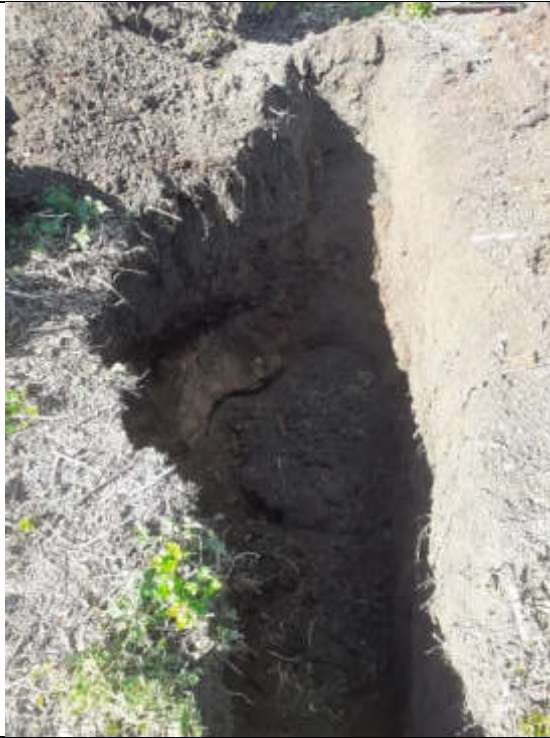
Plate 55: TP107 finished excavation.
