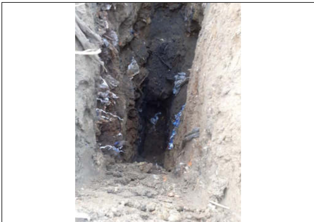
Plate 182: TP122 finished excavation.
