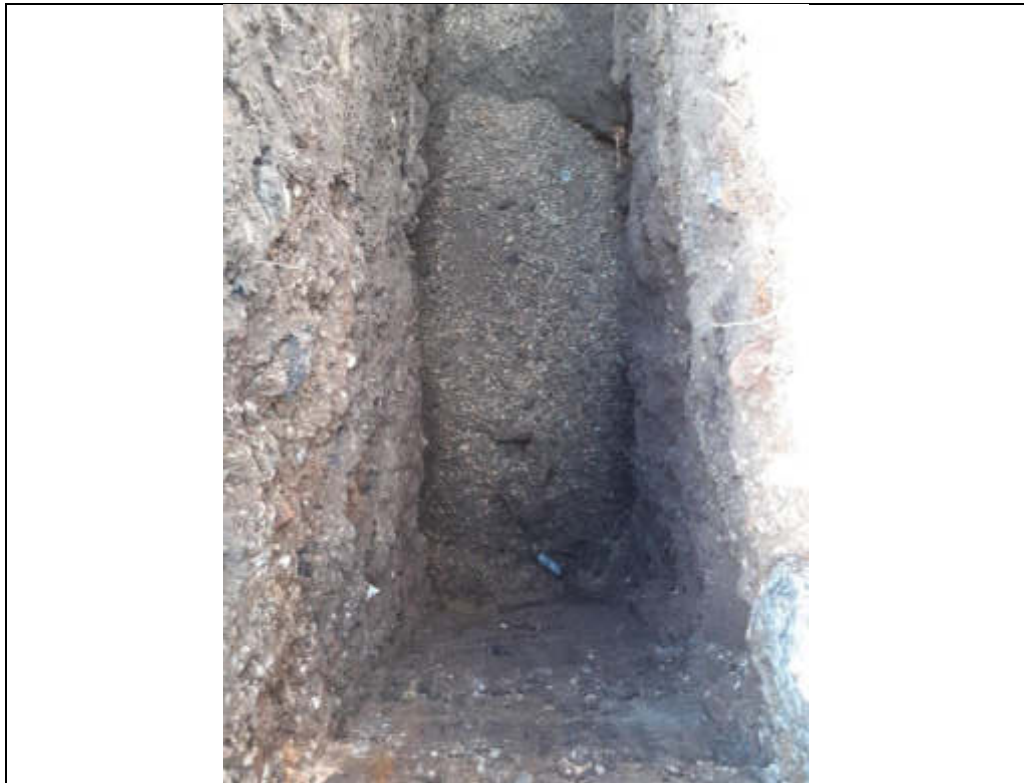
Plate 29: TP104 finished excavation.
