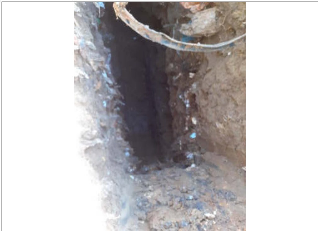
Plate 246: TP128 finished excavation.
