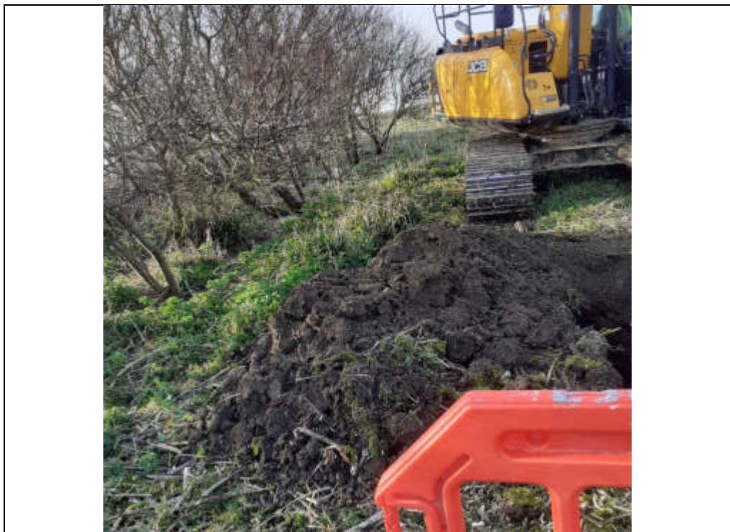
Plate 176: TP122 ranging from ground level to 0.5 m bgl.
