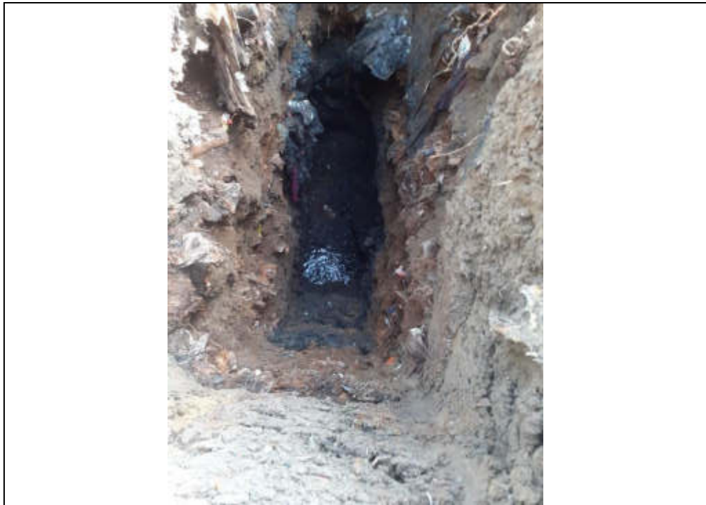
Plate 145: TP118 finished excavation.
