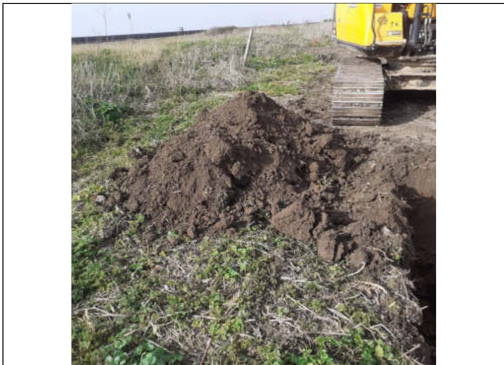
Plate 166: TP121 ranging from ground level to 0.6 m bgl.
