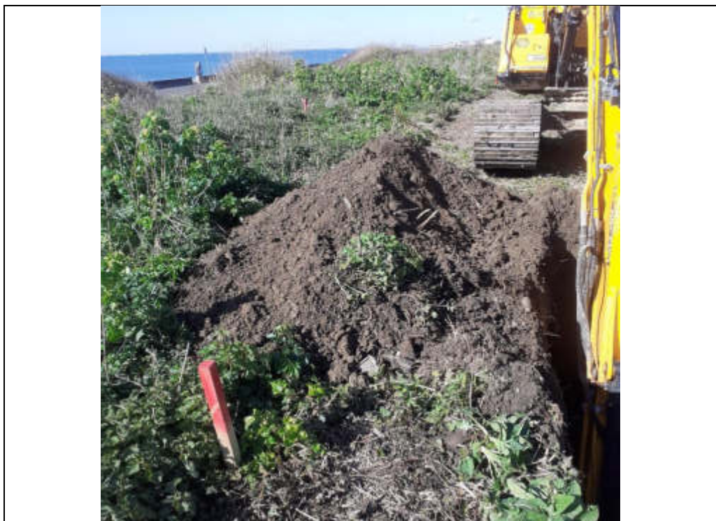
Plate 60: TP108 ranging from ground level to 0.9 m bgl.
