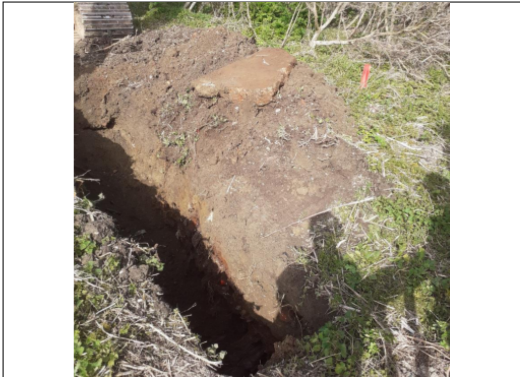
Plate 151: TP119 showing boulder of concrete.
