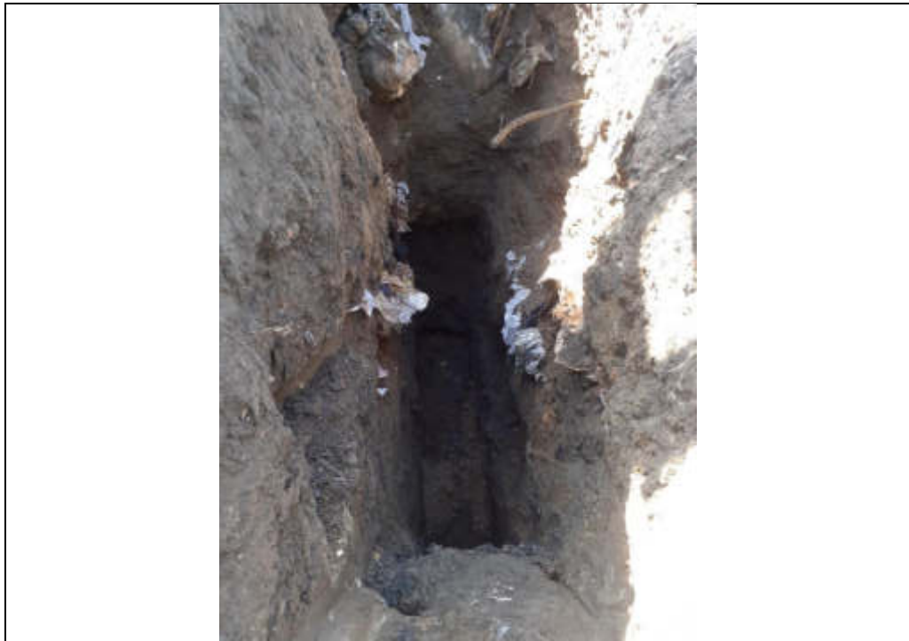
Plate 255: TP129 finished excavation.
