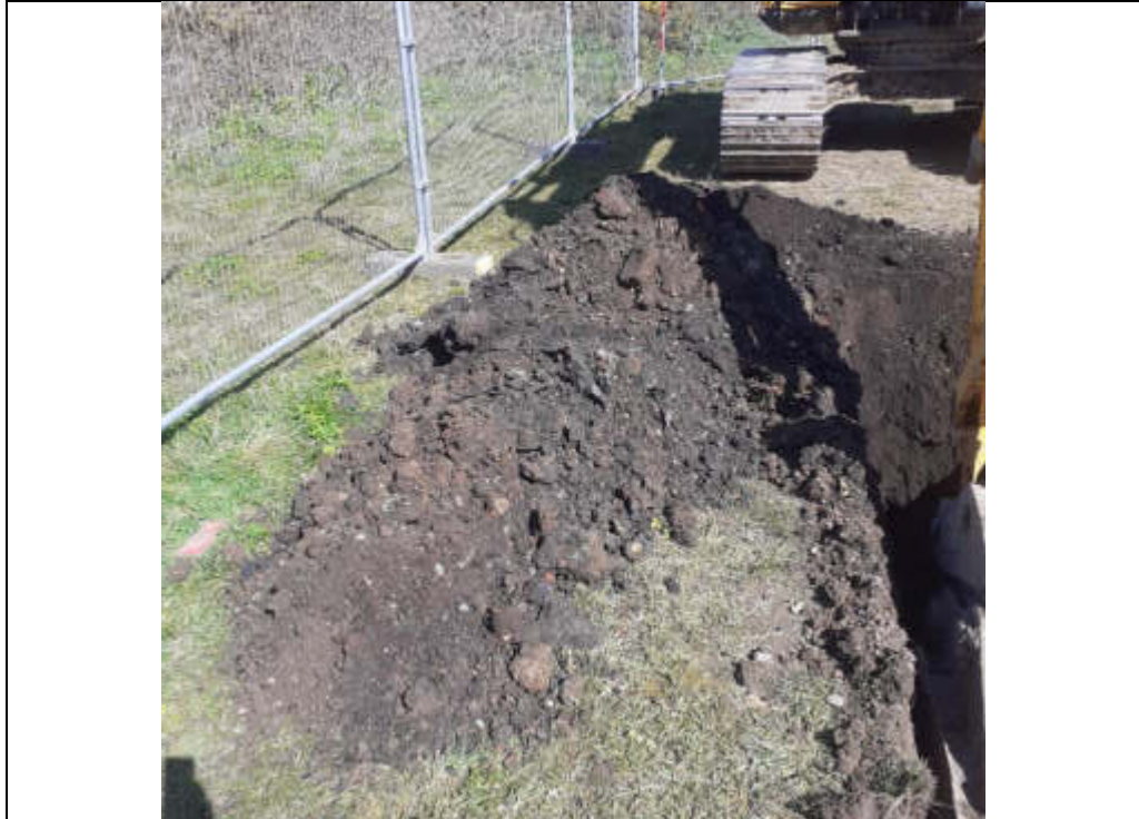
Plate 270: TP131 ranging from ground level to 0.4 m bgl.
