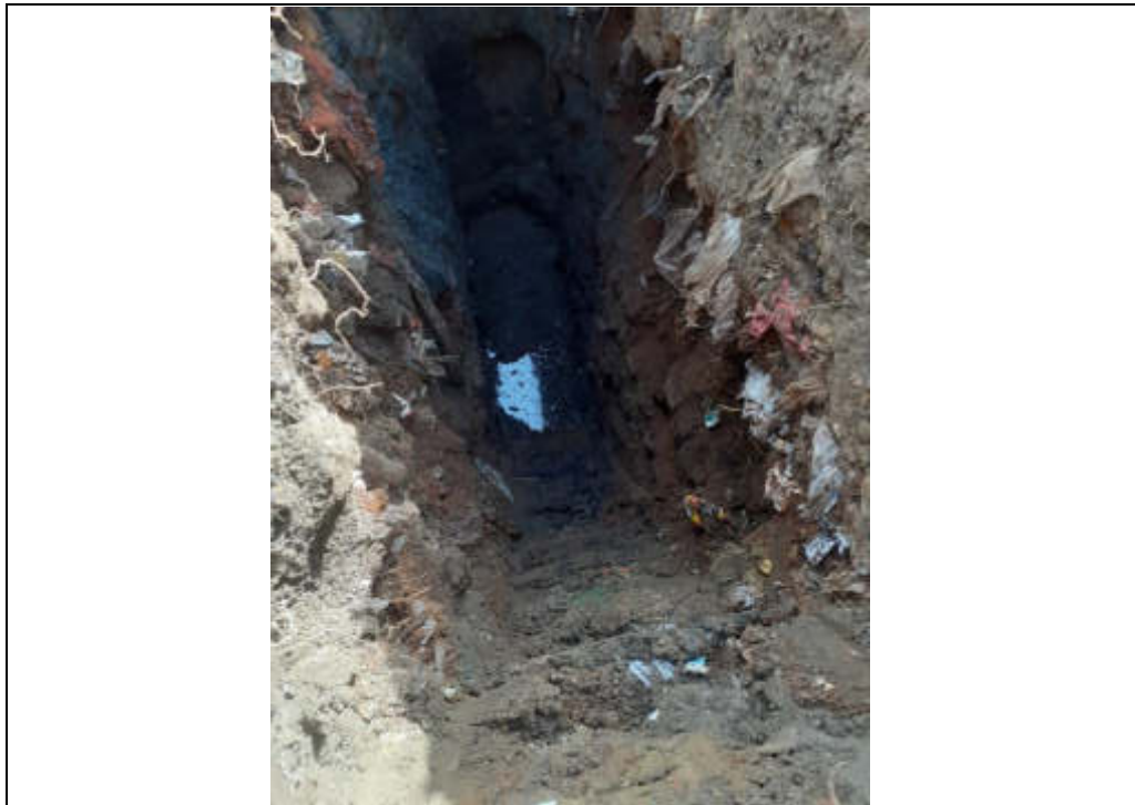
Plate 161: TP120 finished excavation.
