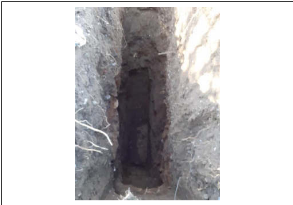
Plate 72: TP109 finished excavation.
