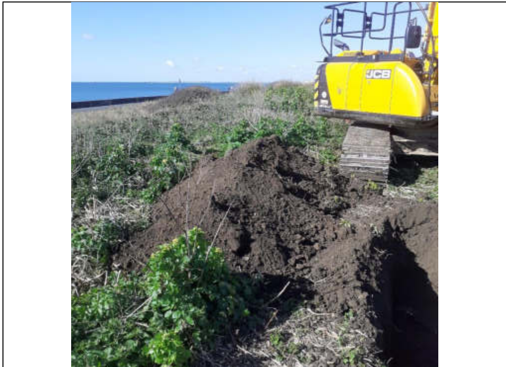
Plate 63: TP108 ranging from ground level to 0.9 m bgl.
