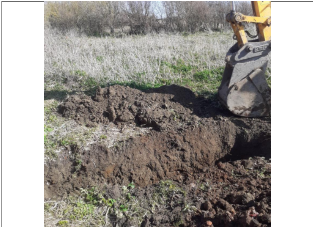
Plate 188: TP123 ranging from ground level to 0.5 m bgl.
