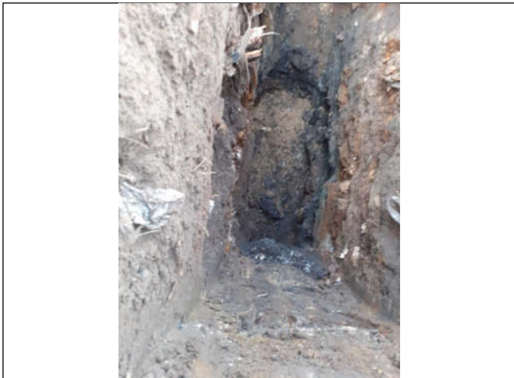
Plate 170: TP121 finished excavation.
