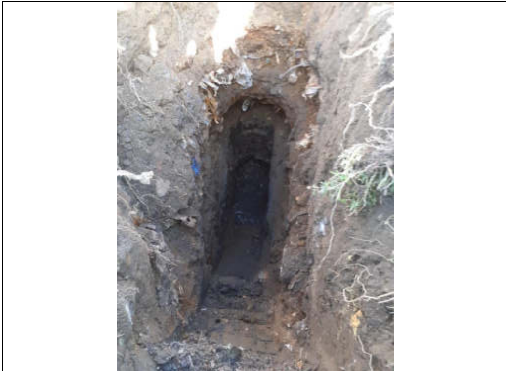
Plate 213: TP125A finished excavation.
