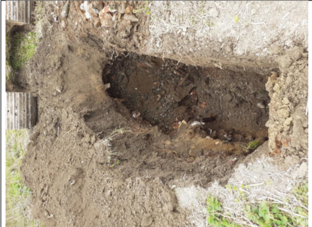
Plate 127: TP116 finished excavation.
