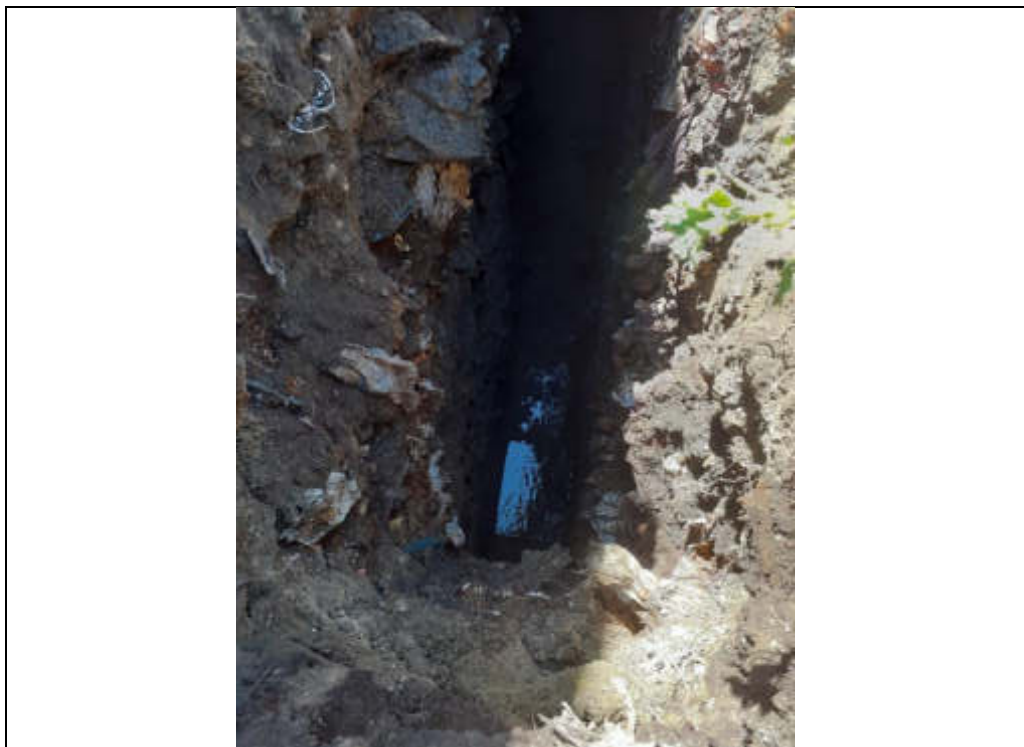
Plate 264: TP130 finished excavation.
