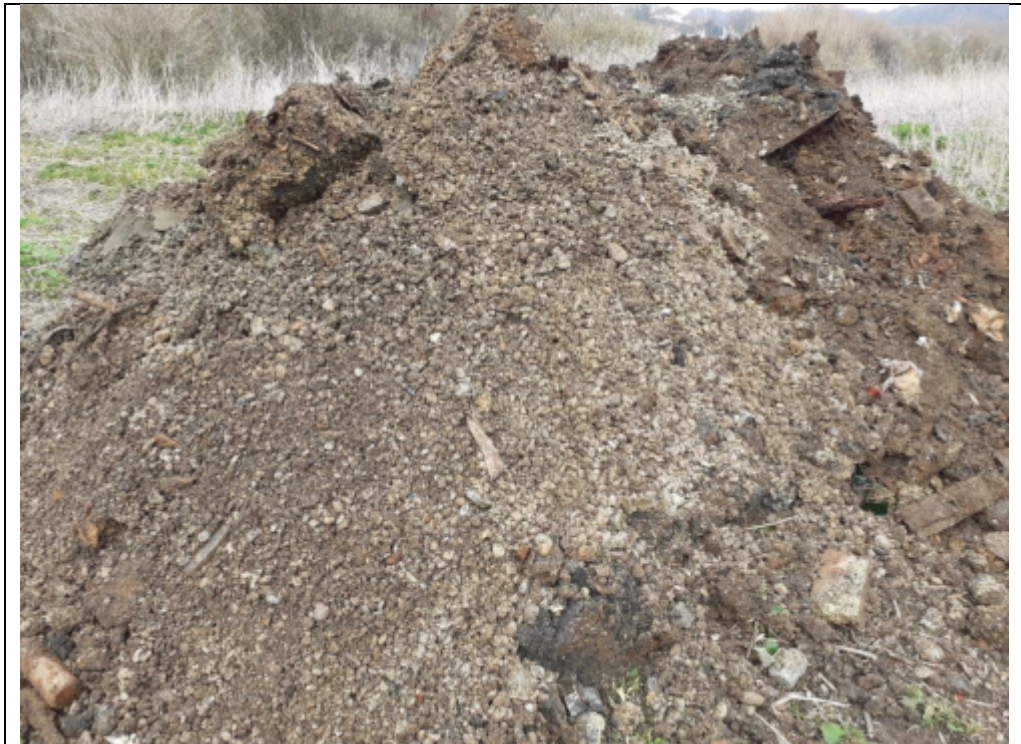
Plate 137: TP117 showing final stockpile.
