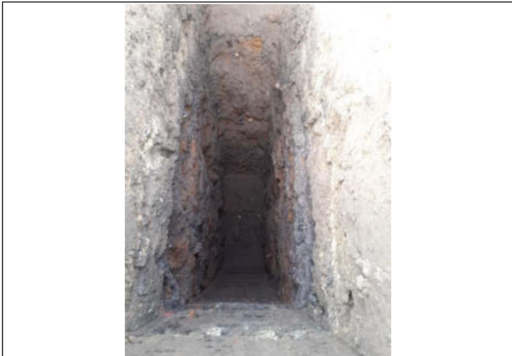
Plate 22: TP103 finished excavation.
