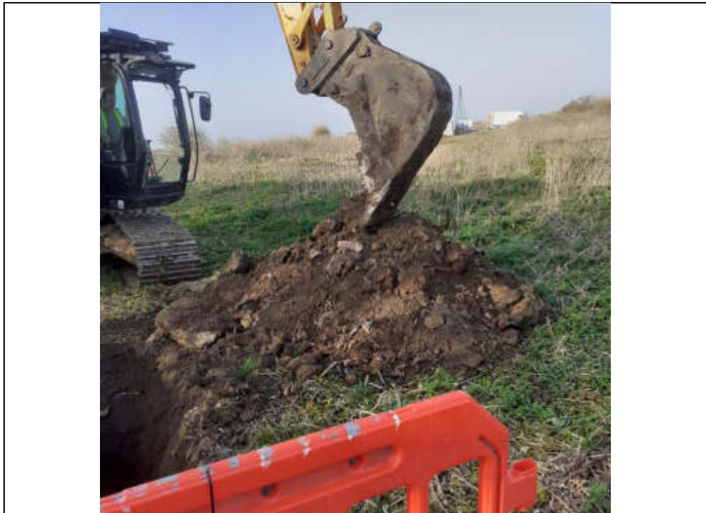
Plate 177: TP122 ranging from 0.5 to 3.3 m bgl.
