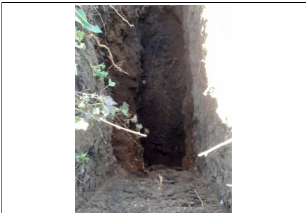
Plate 64: TP108 finished excavation.
