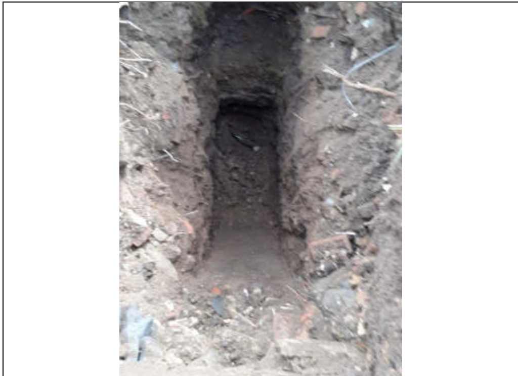
Plate 15: TP102 finished excavation.
