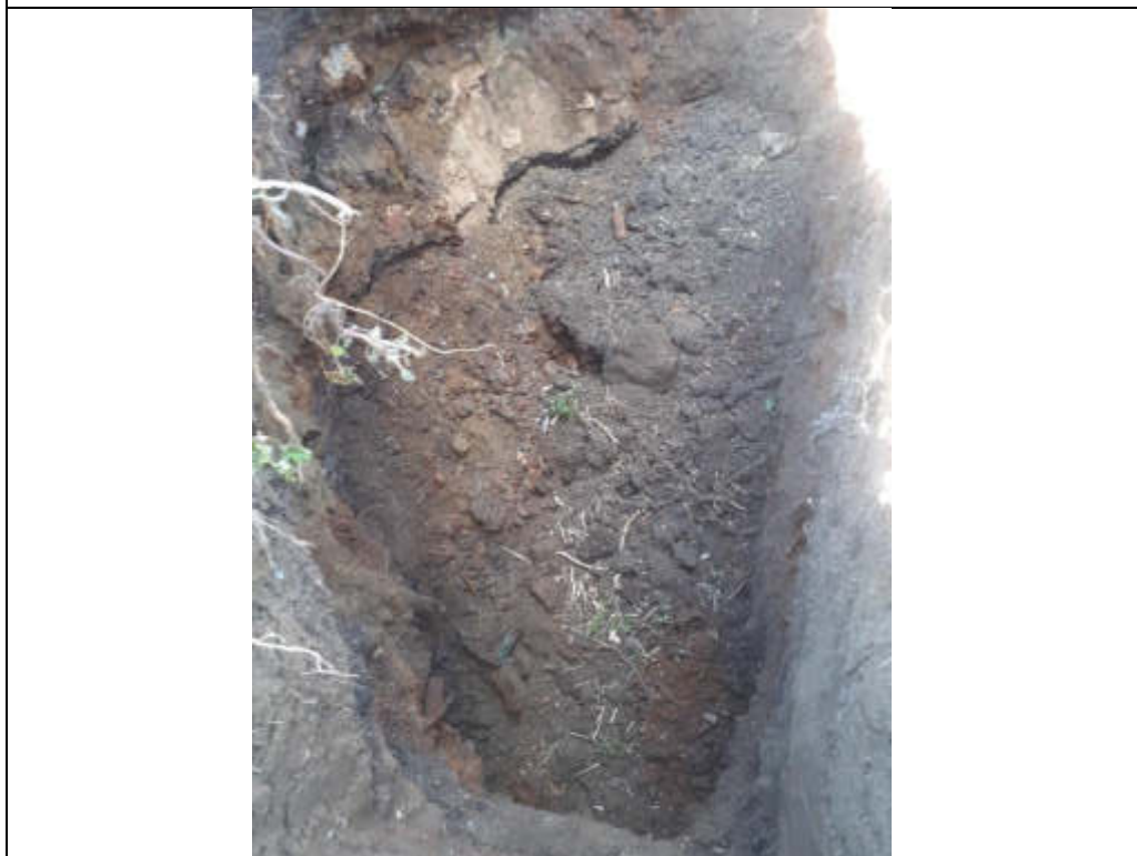
Plate 54: TP107 showing pit collapse.
