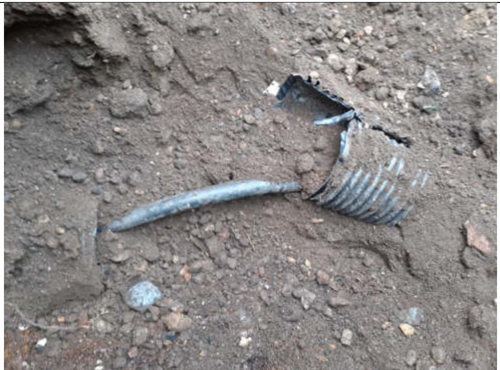
Plate 04: TP101 – electricity cable identified within plastic ducting at 0.9 m bgl.
