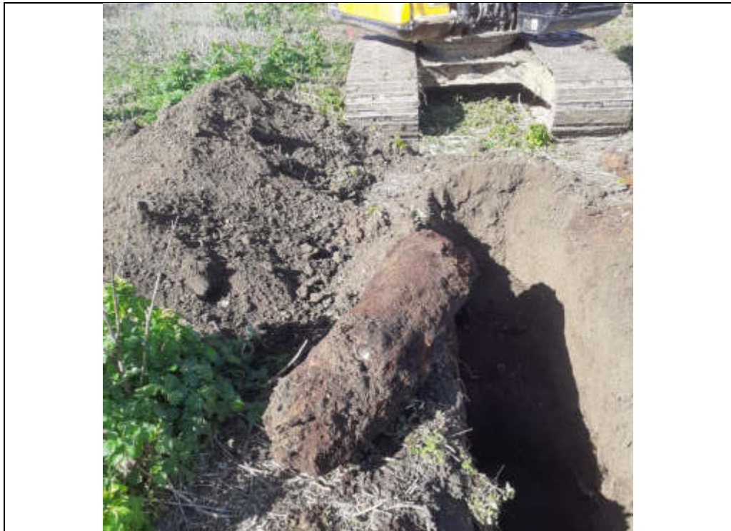
Plate 53: TP107 – wooden log identify at 2.0 m bgl.
