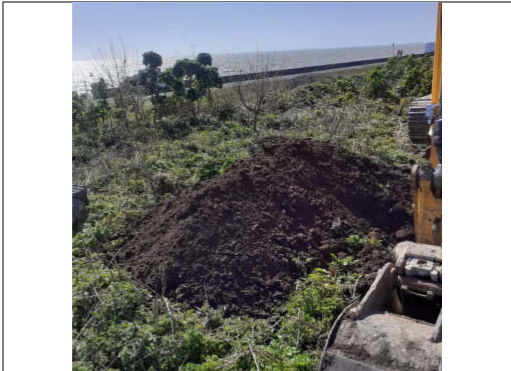
Plate 251: TP129 ranging from ground level to 1.0 m bgl.
