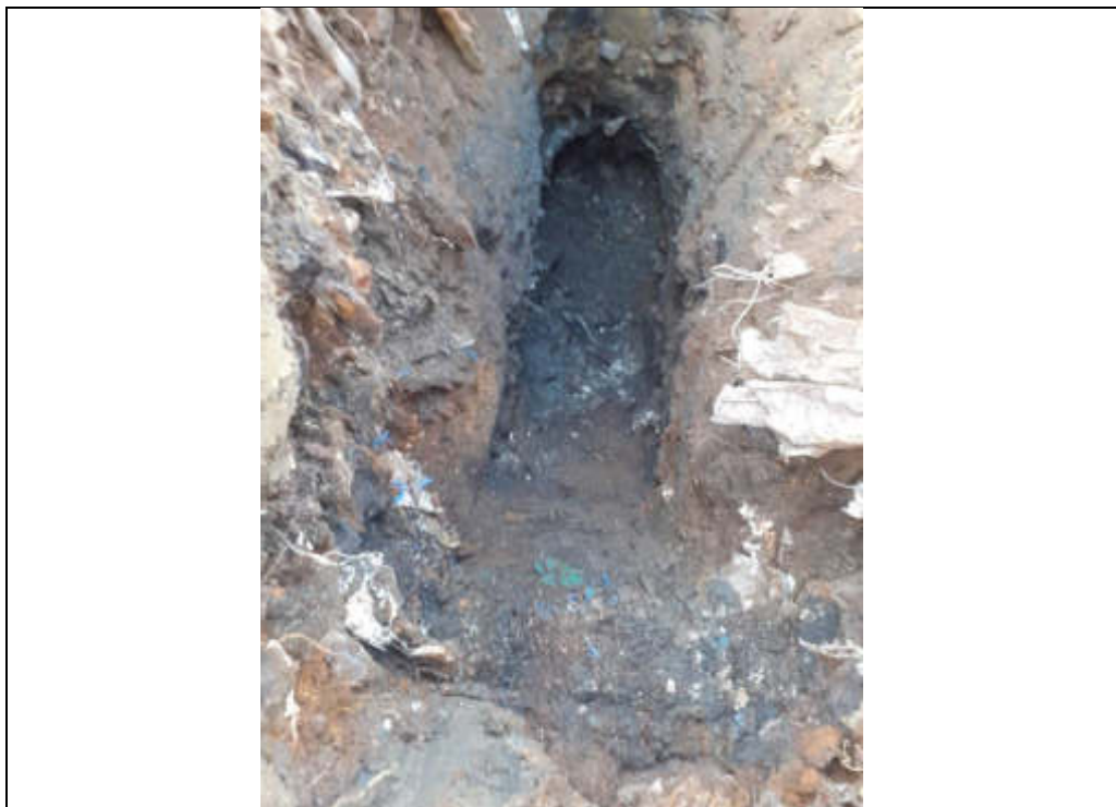
Plate 154: TP119 finished excavation.
