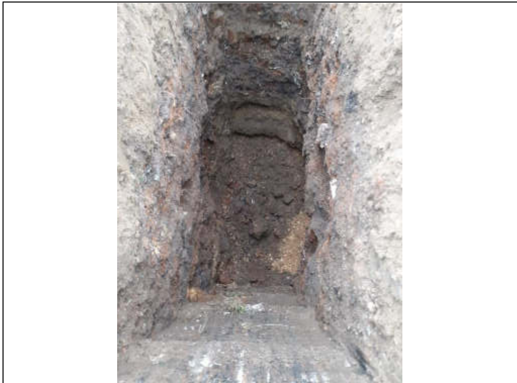
Plate 07: TP101 finished excavation.
