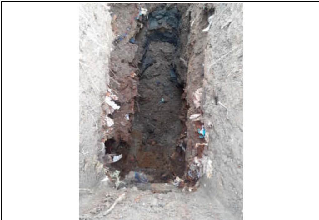
Plate 138: TP117 finished excavation.
